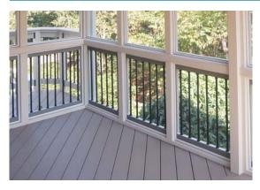
Figure 6. Elevated porches — even when screened — require guards to prevent falls.
