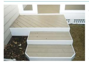
Figure 5. Porch flooring raised slightly above an abutting deck helps keep out water. This detail should only be done where traffic enters through a door, so that occupants are clued in to the elevation change.
