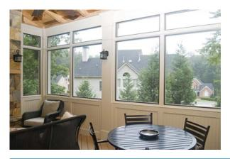
Figure 7. Kneewalls provide guards, privacy, and a place for electrical outlets.
