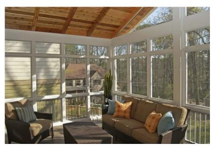
Figure 8. Timber rafters that stack atop the posts provide a clear load path. Tongue-and-groove 2-bys above provide both a finished ceiling and a roof deck.
