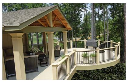
Figure 10. Open porches have fewer posts than screened porches. To maintain the look of adequate support, the author wraps such posts with trim to increase their width.
