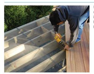
Figure 4. Screening under the decking helps prevent bug invasions from below.
