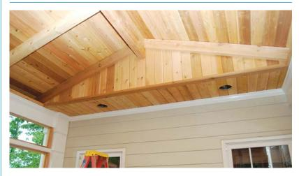
Figure 2. Covering a house's second-story cantilever with the same material that's on the porch ceiling helps to blend it in.
